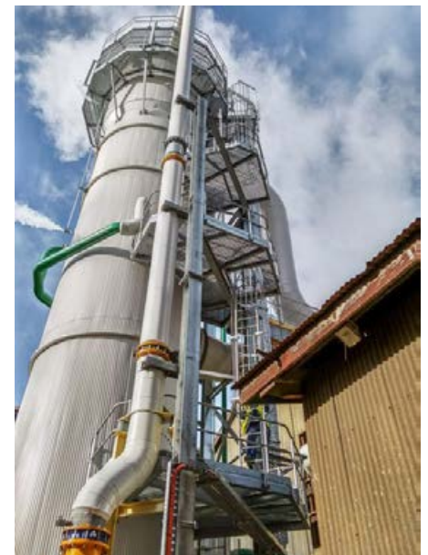
Falling-film tube evaporator at the Bingera Mill
