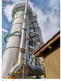
Falling-film tube evaporator at the Bingera Mill
